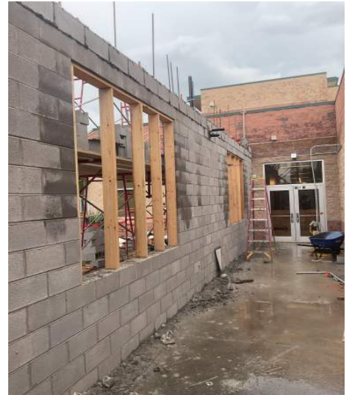
CMU Load Bearing Wall
